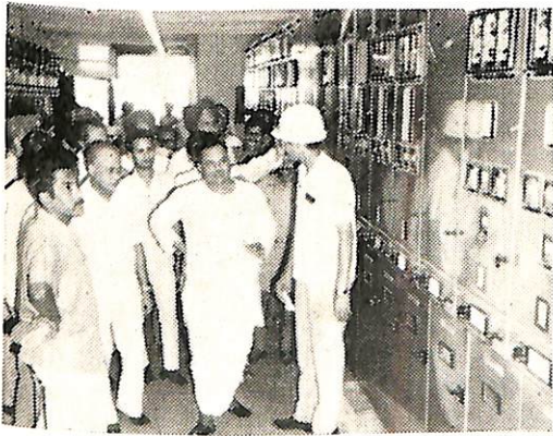
Shri D. L. Sekhar Deo, Minister of State for Irrigation and Power going round the main Power Station of the Talcher Fertiliser Plant after switching on the power line
